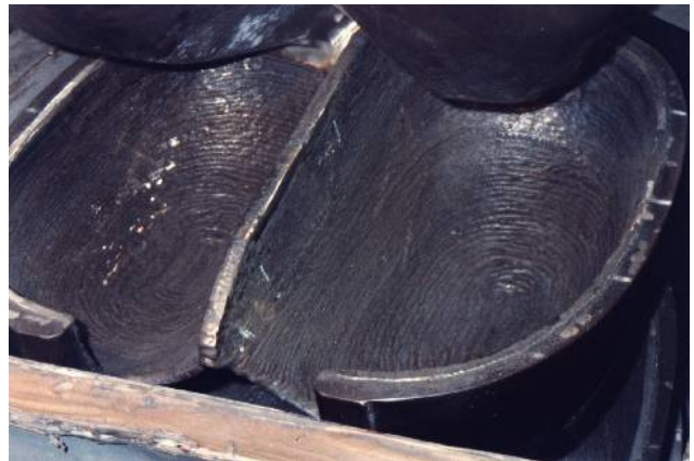
Fig. 1 – TIG welding of the buckets
