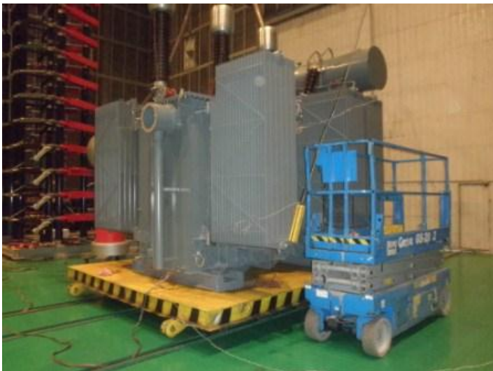
Transformer during the FAT tests
