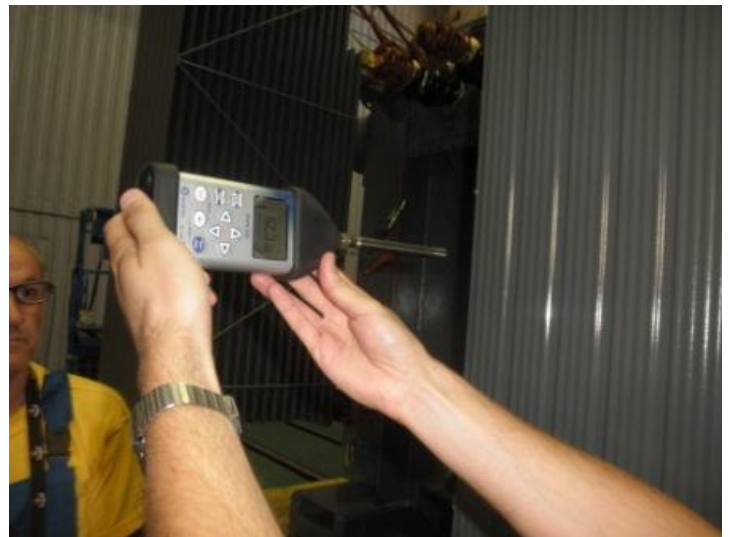
During FAT test: Measuring the sound level at 0,3 mts
