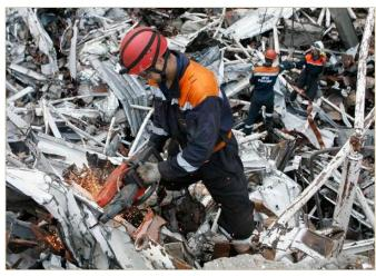
A large quantity of water coming from the Yenisei River knocked down the turbines hall, provoking the <u>explosion of at least one transformer. All the turbines were badly damaged.</u> 75 people were killed during this accident.
