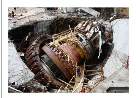
The report identified the cause of the accident to be a bolt failure in the cover of one turbine, due to vibrations. 49 bolts retrieved after the accident were tested and fatigue cracks were detected on 41 of them.
