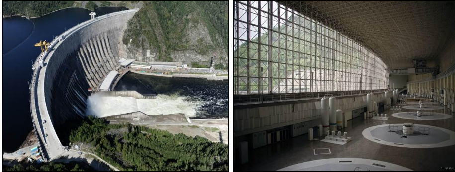
Figure 7. Sayano-Shushenskaya plant, before the accident
