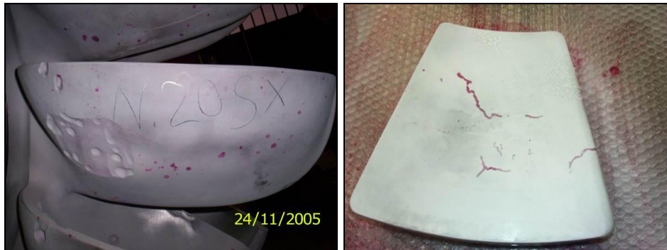
Figure 2. Example of defects on a Pelton runner and white metal bearing segments detected during a Liquid Penetrant examination
